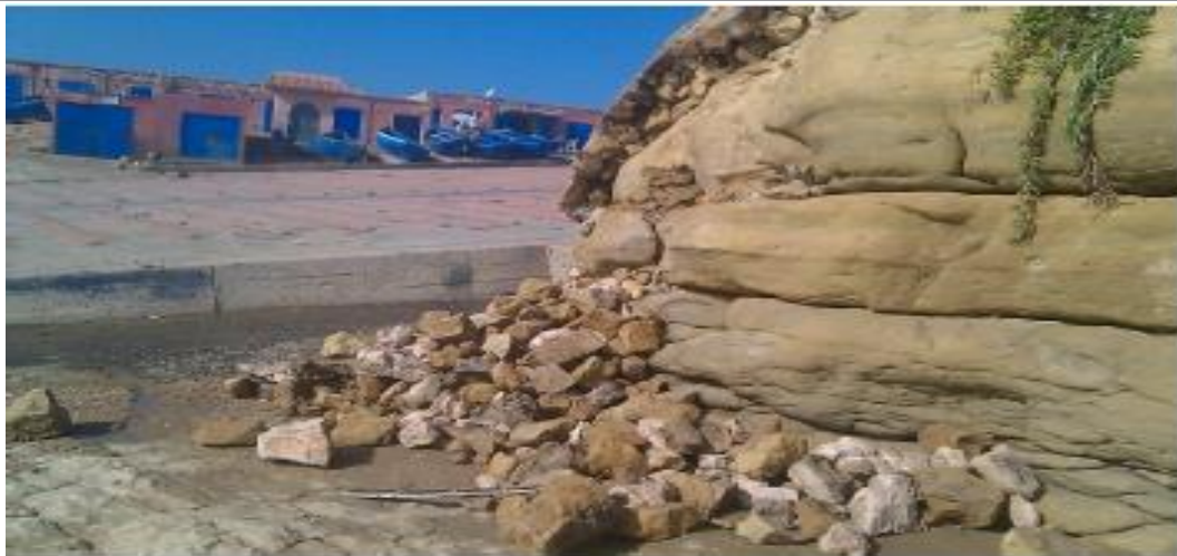
Figure 27: Destruction du mur e dallage
